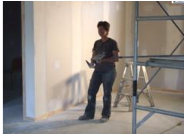
Gib-Stopping completed – Val Lowe in Action.
